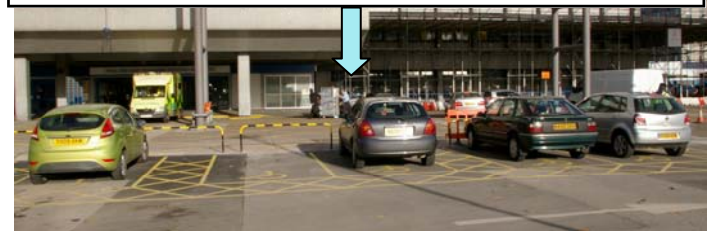
New Disabled Car Parking Bays
